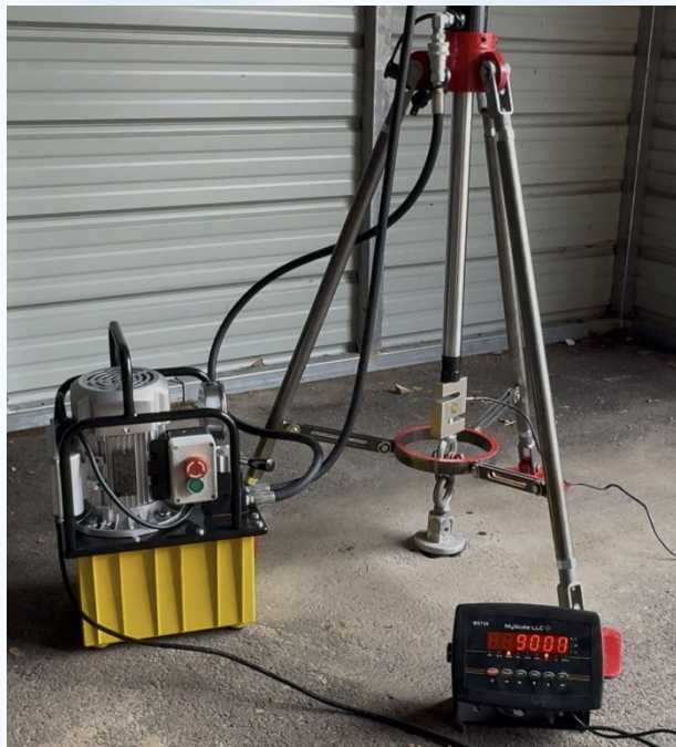
Figure 11: Proof load of a PE36-Hex in asphalt pulling at 9,000 lbs using an optional load cell
