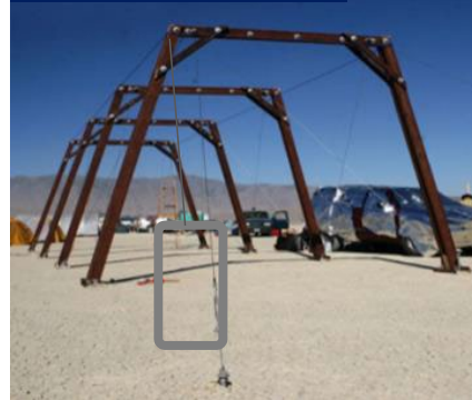
PE26 with tie-off cable to turnbuckle
