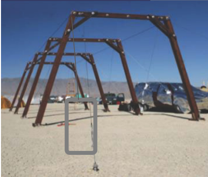
PE26 with tie-off cable to turnbuckle
