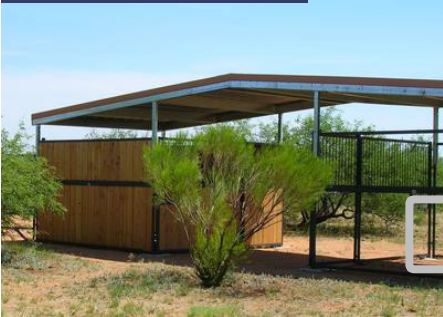
PE18 with tie-off cable up to a fitting on shelter's leg
