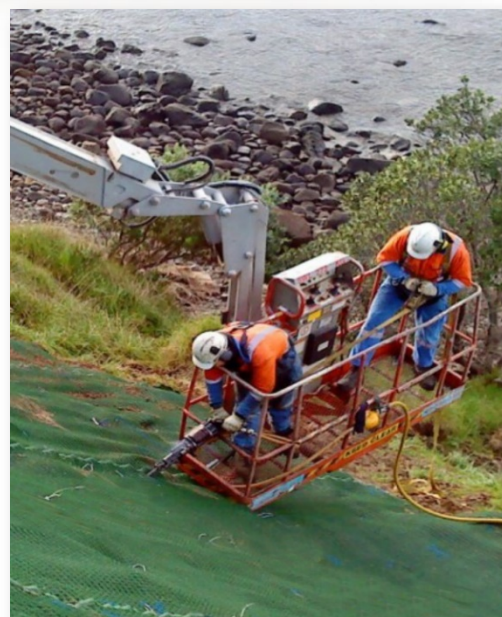
Driving anchors into hillside using hammer drill
