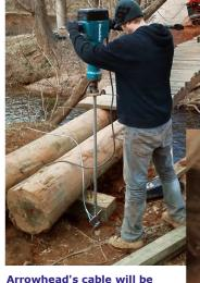
Arrowhead's cable will be wrapped around the horizontal logs, using a large loop held with cable clamps
