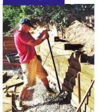
Another locking method Wrap cable around the drive rod and pull
