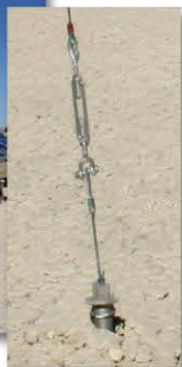
Hardpan method: Drill 1" x 10" pilot hole
