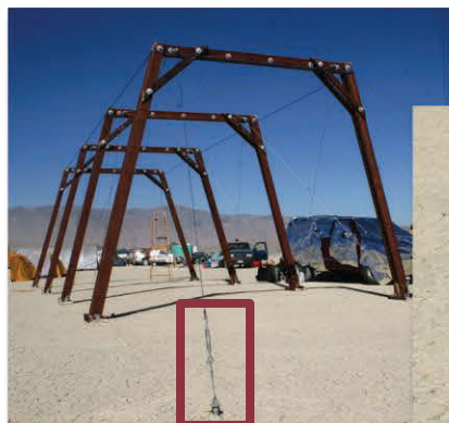
PE26 with tie-off cable to turnbuckle
