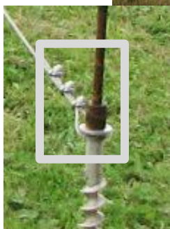
Cable clamps for guy-wire's loop around PE26
