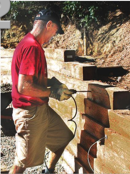
Drill hole and pass the cable out through it
