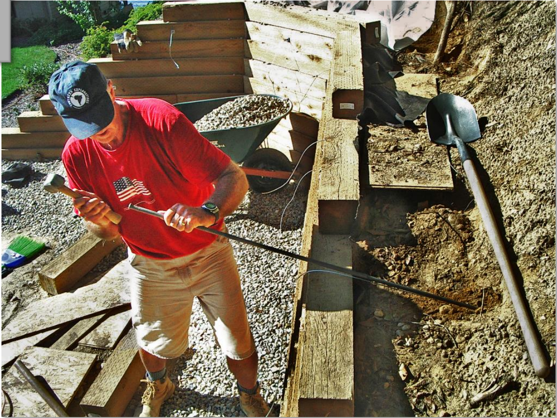
Drive in the anchor
