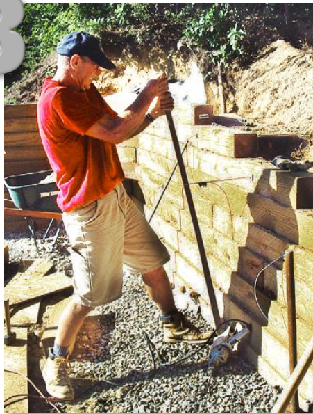
Pull to lock the anchor Common pulling method is cable wrapped around the drive rod
