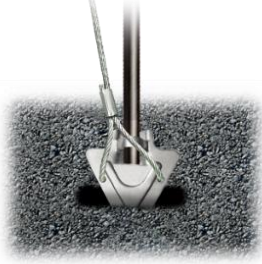
One method: Jackhammer with chisel
