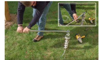
TIP: Add a steel pipe to the handle of a ratchet wrench for leverage.
