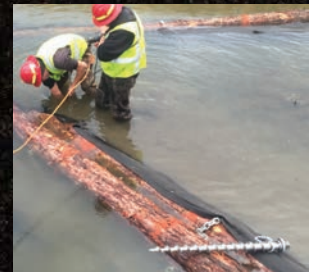
Log Cabling / Erosion Control
