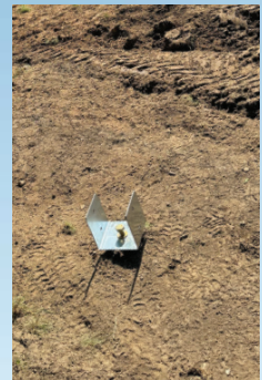
UBracket Bolted to PE46-Flat
