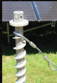
Tie Off Cables
