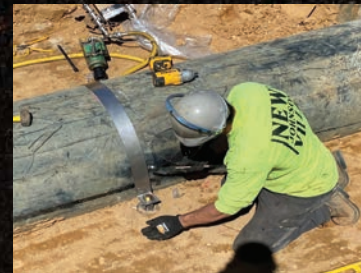
Custom Strapping. Shown here connected to top of anchor with 3/4"-10 bolt.
