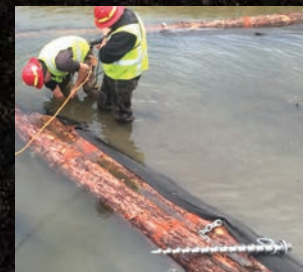
Log Cabling / Erosion Control
