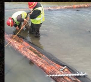
Log Cabling / Erosion Control
