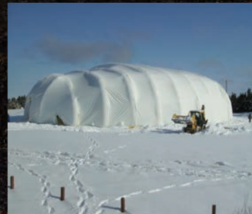
Fabric Shelter in Canada
