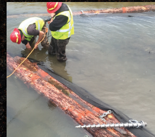
Log Cabling / Erosion Control
