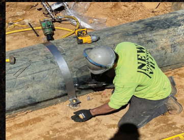
Custom Strapping. Shown here connected to top of anchor with 3/4"-10 bolt.
