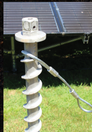
Tie Off Cables
